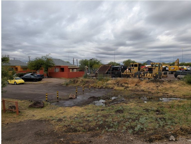
Looking north across the alley, May 5, 2026 at 7:02 AM. Single-family homes (left) sit ~60 feet from the proposed tower base. Yellow bollards delineate the regulatory wash; behind the fence: a CAT excavator, graders, stacked drainage culverts. EXIF GPS preserved.
